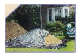
This picture of the contaminated soil from a leaking underground storage tank includes the covering over the soil to prevent further contamination during cleanup. This soil will be placed in a landfill certified for petroleum contaminated soil.
