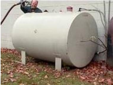
Make sure your tank has an over-fill protection detection device installed to prevent accidental spills. Many tanks have an inexpensive alarm installed to prevent overfills, or use a measuring gauge on the side of the tank to show the level of the fluid in the tank. Supervise the delivery and transfer of fluid into the tank to make sure that all precautions are taken.
