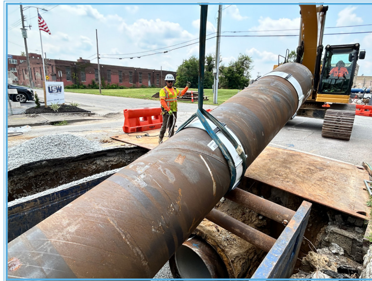
Louisville Water is replacing a 130-year-old water main.
