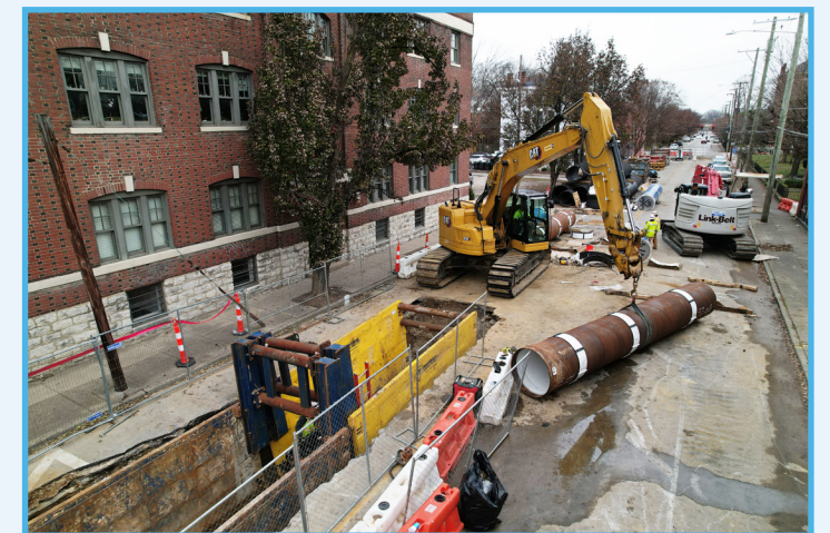
Crews are replacing a 130-year-old, 48” transmission main along Oak Street
